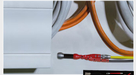
Shafts and underfloor ducting
