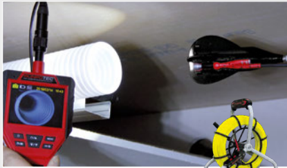
Ventilation inspection and servicing
